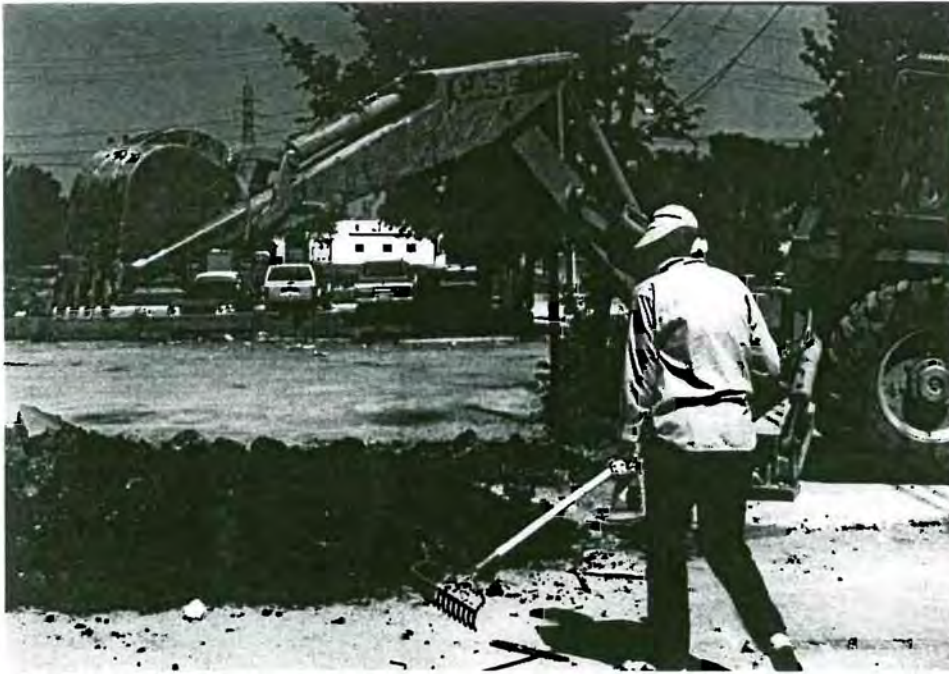
Plate 3: Backhoe dumping a bucket of excavated soil.
