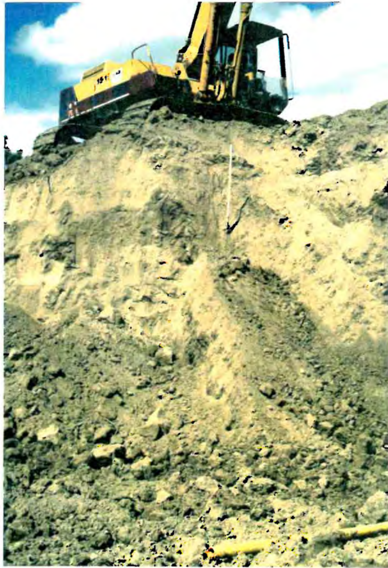
Plate 2: Vertical Excavation Wall at South Abutment
