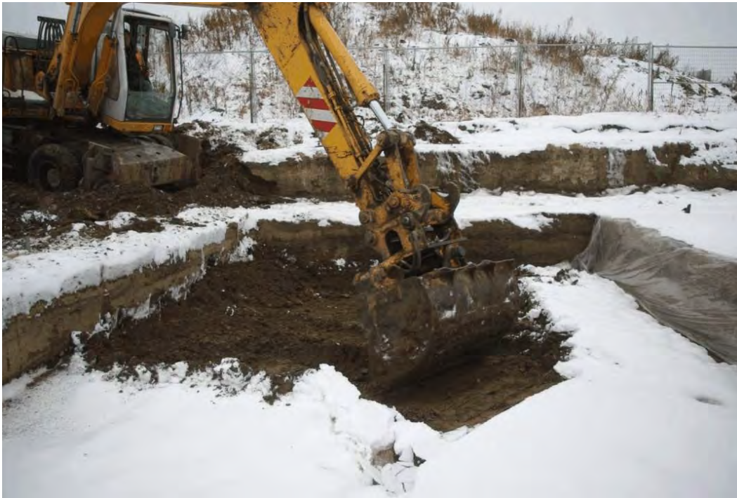
Plate 1.5-3: Large Backhoe with Ditching Bucket to Excavate Exploratory Hole
