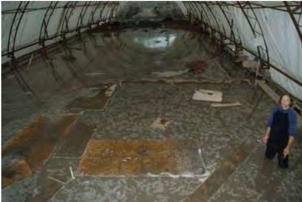
Plate 1.3-2: Excavation Area After First June 27 Flood
