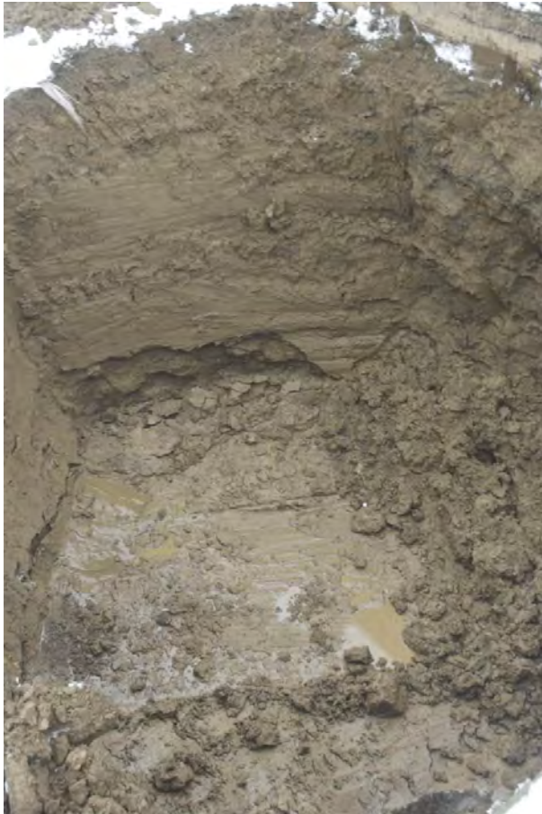
Plate 1.5-4: Water Seepage at Base of Hole
