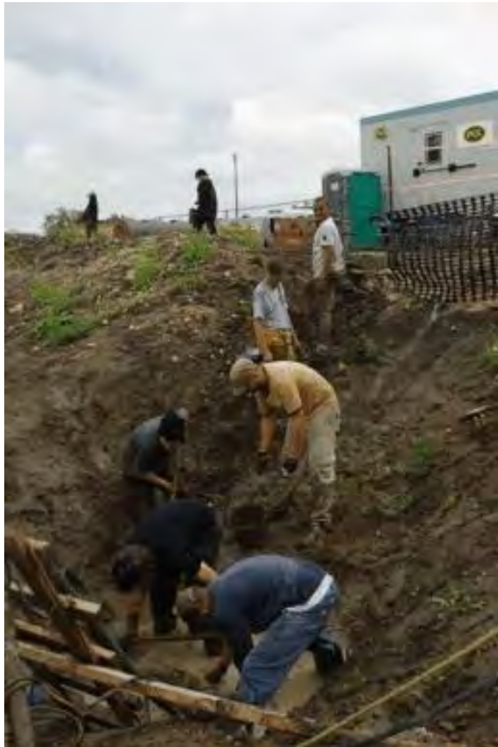
Plate 1.3-3: Crew Cleaning Sump Pit after a Deluge
