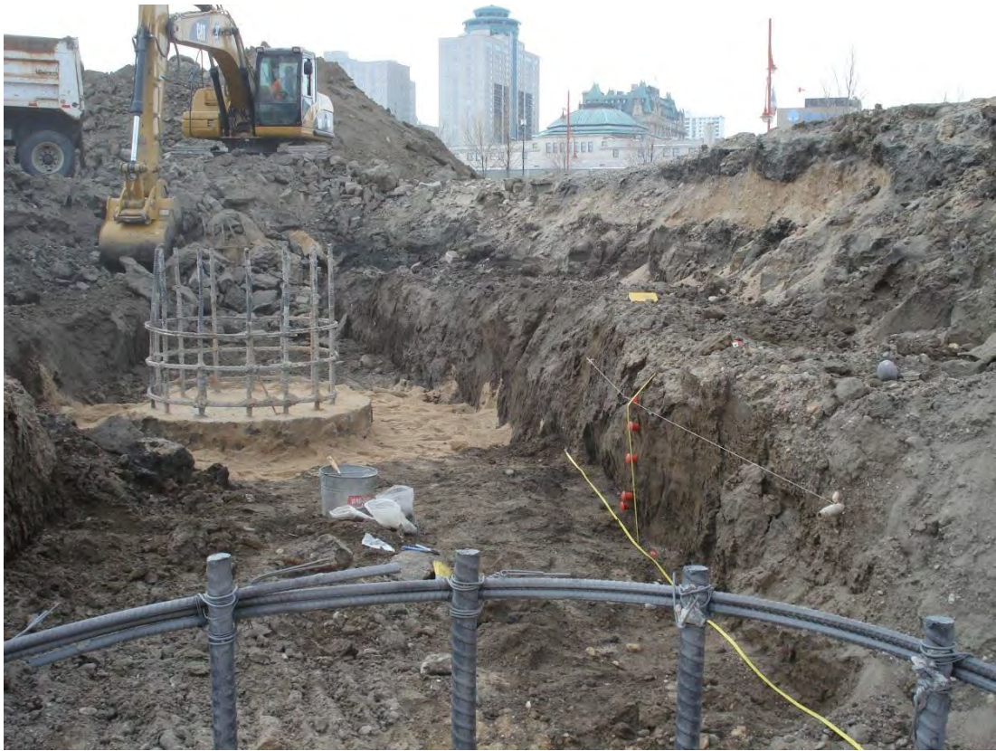
Photo 15-15: Grade beam excavations and archaeological recording in progress in Root C.
