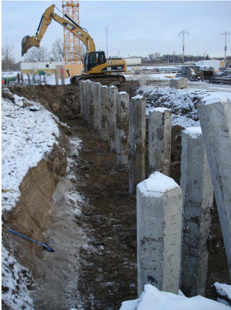
Photo 15-16: Grade beam excavations in northeast corner of Root D.
