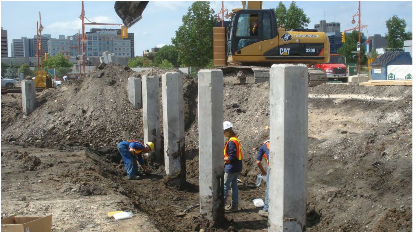
Photo 15-10: Configuration of precast piles in northwest corner of Root A
