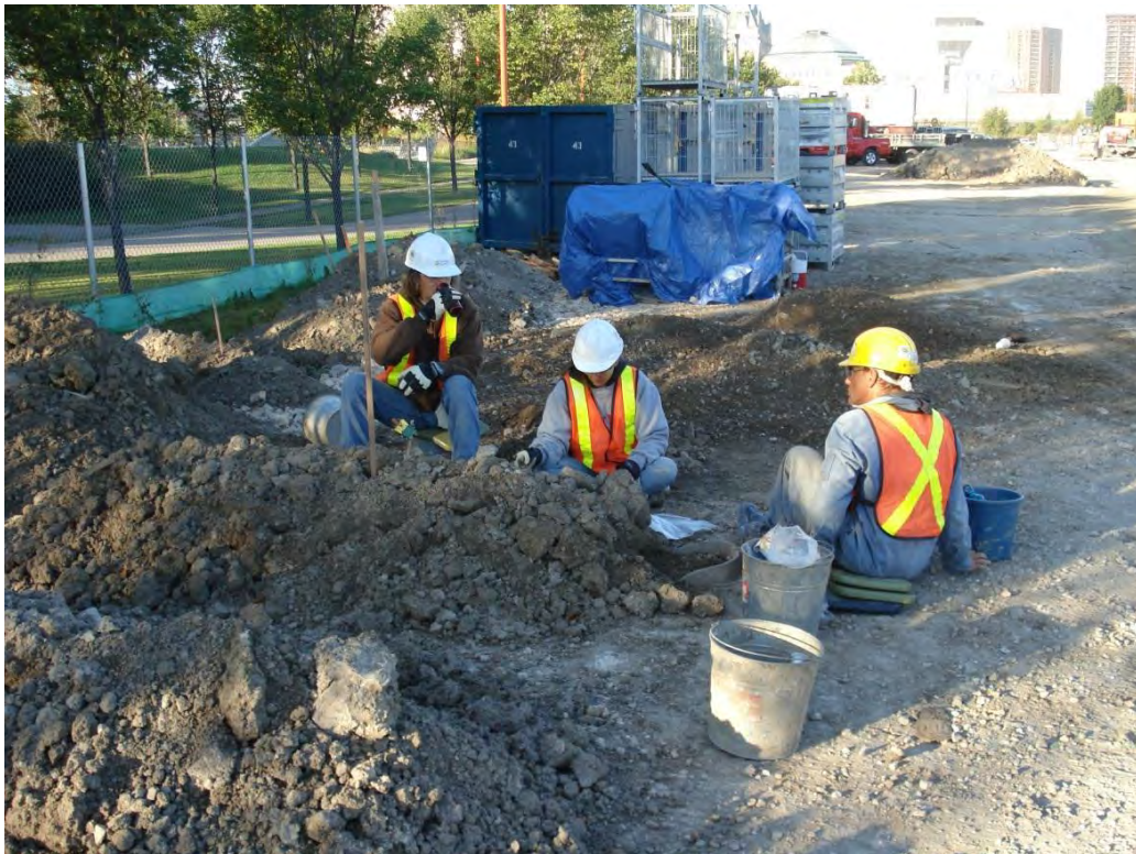
Photo 15-6: Hand screening spin-off piles at edge of CMHR property.
