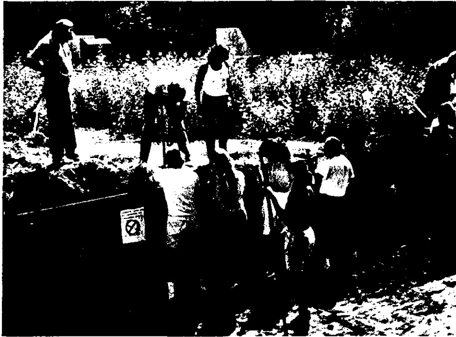
Figure 5: Installing Shoring in the 1990 Extension
