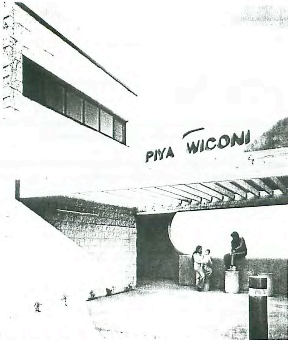
Piya Wiconi: deck separating caretaker's flat from the main community building.
