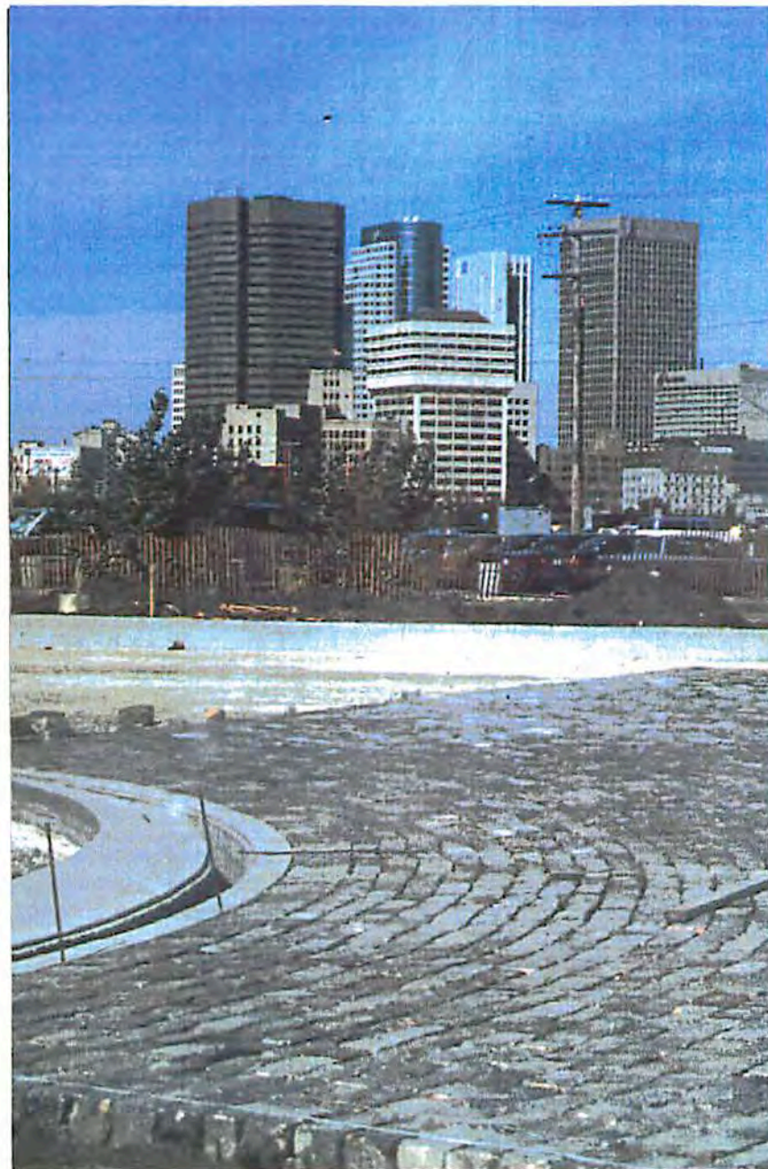
The cobblestone cul-de-sac (under construction) will terminate historic Portage Trail.
