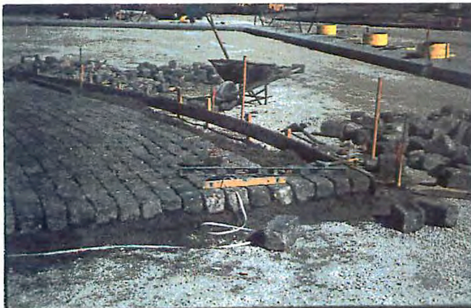
Detail of cobblestone paver installation.
