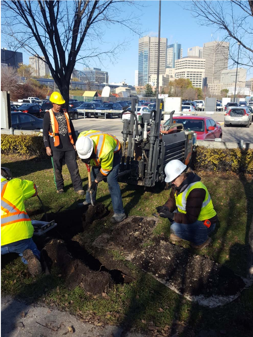
Figure 8: Examining Excavated Soils from Trench
